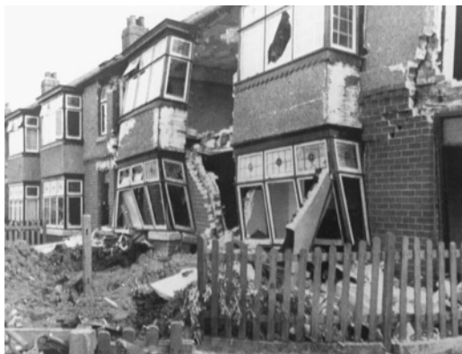
War damaged houses
